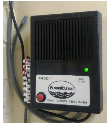
Figure 2 - Leak Detection System
