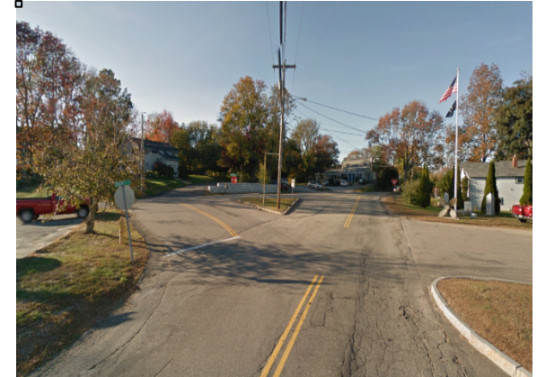
Intersection of State Road and Rogers Road, one of the high crash locations.
