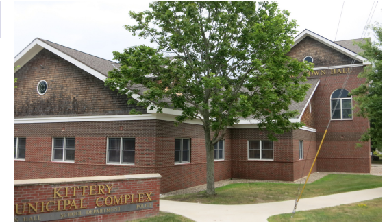
The Municipal Complex houses the majority of the Town's administrative offices.
