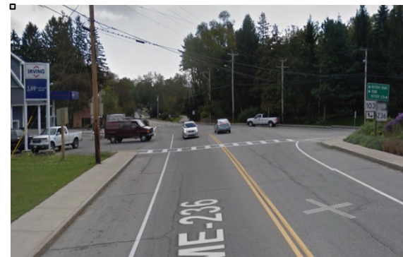
Unsignalized intersection of Shapleigh Road/Whipple Road/Woodlawn Avenue
