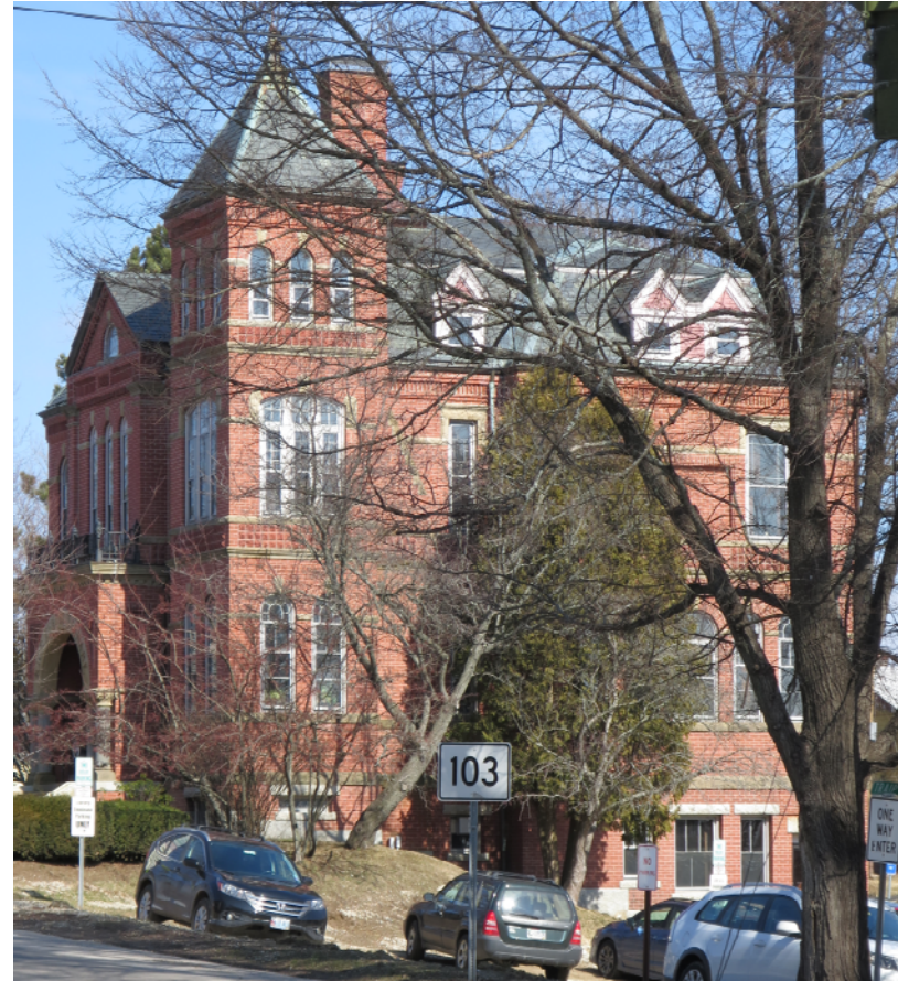
The Rice Public Library, located on Route 103 in Kittery Foreside, is one of the town's most prominent historic structures and a centerpiece of the historic Foreside area.
