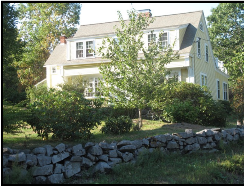
A typical older single-family home in Kittery.
