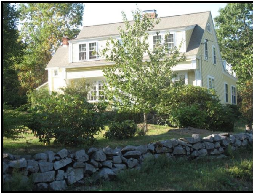
A typical older single-family home in Kittery.
