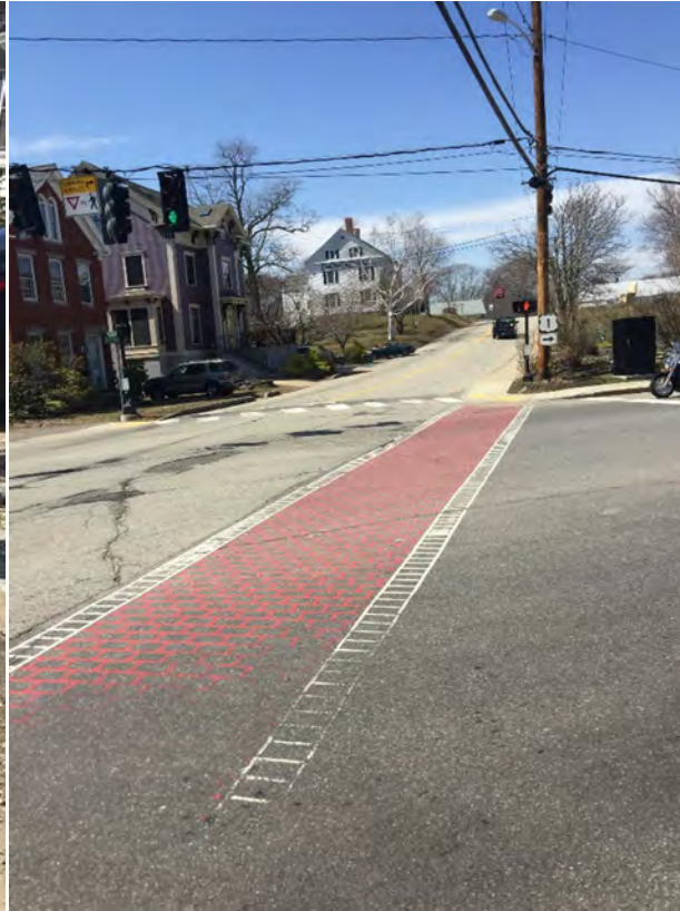
Crosswalk paint is fading and hard to see in some locations.
