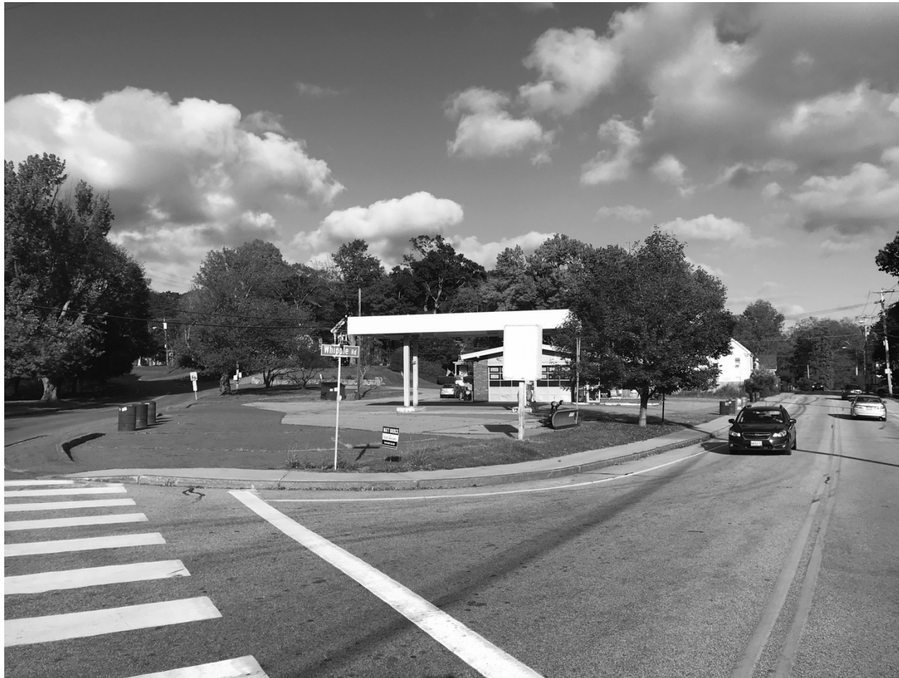
Figure 52 – Existing Conditions at Wentworth and Whipple
