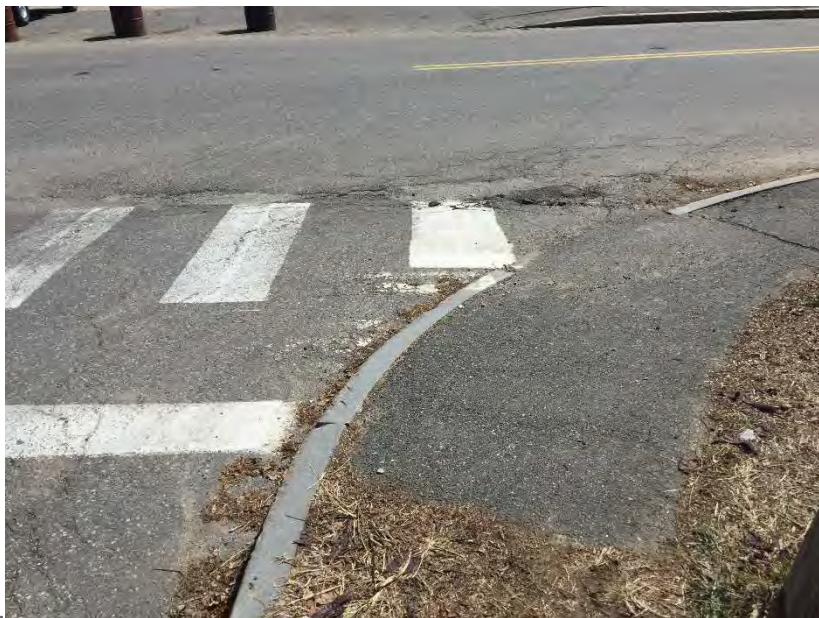
Non-compliant ADA conditions and marking visibility.
