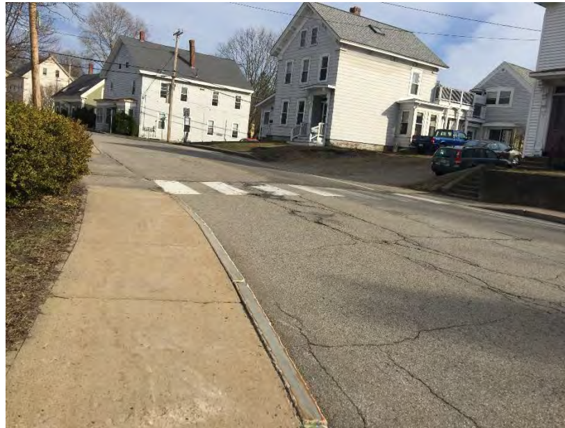
Limited sight visibility at mid-block crossing and ADA compliance.
