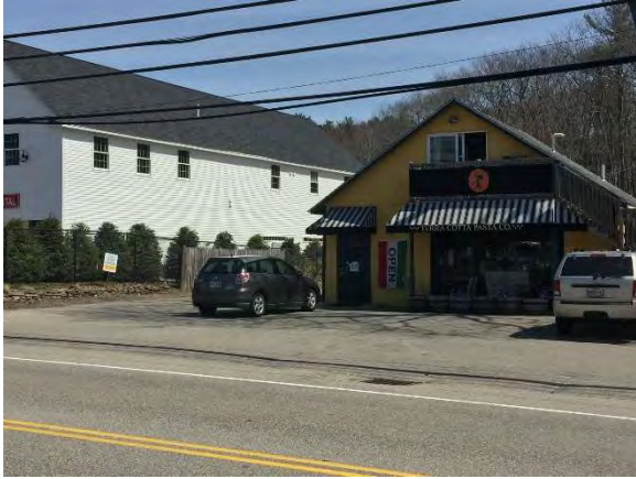
Wide driveway opening creates unsafe crossing.
