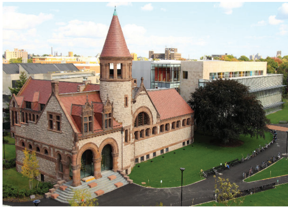
Honor Historically Significant Structures
