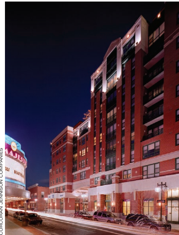
Corcoran Jennison's Park Square West luxury apartment development in Stamford, Connecticut, reserves 20 percent of the units as affordable. Low-income housing tax credits were allocated for the affordable units.
