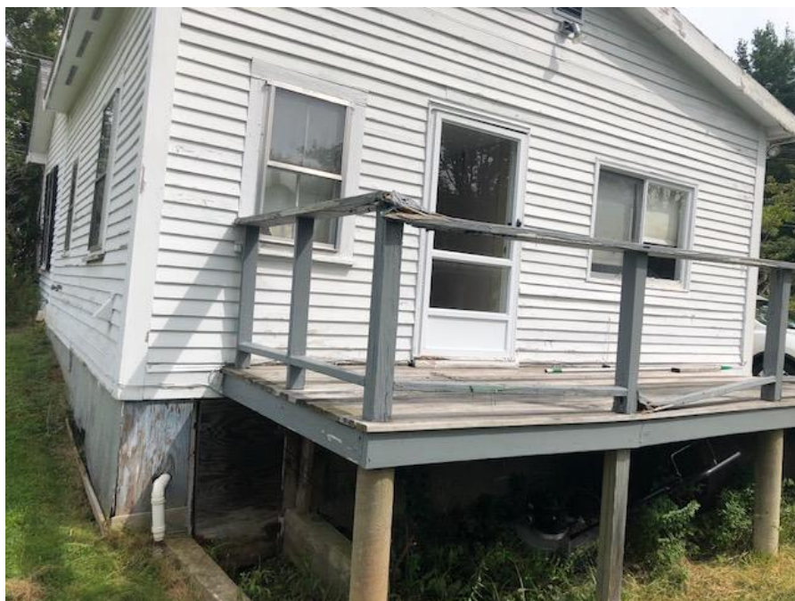
BACK OF BUILDING
