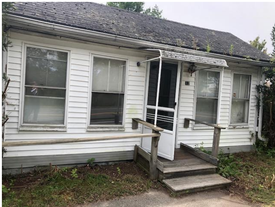
FRONT OF BUILDING
