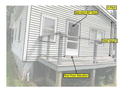
Based upon a combination of the data collected in the field and the data generated using the old photos, the horizontal and vertical dimensions of the existing structure were established. An elevation view of the back of the building that labels key dimensions and elevations is provided on the revised Shoreland Development Plan.
