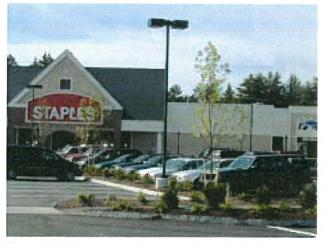
These light fixtures have been coordinated with the planting plan to avoid problems as the trees mature. Slightly raised bases protect the poles from plow damage.
