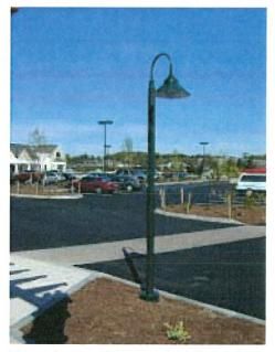
This pedestrian fixture has been located to illuminate the crosswalk that leads into a commercial establishment.
