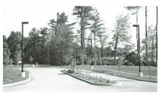
This curbed, landscaped island divides entering and exiting traffic. The identification sign is located away from the intersection to avoid interfering with the motorists' line of sight.
