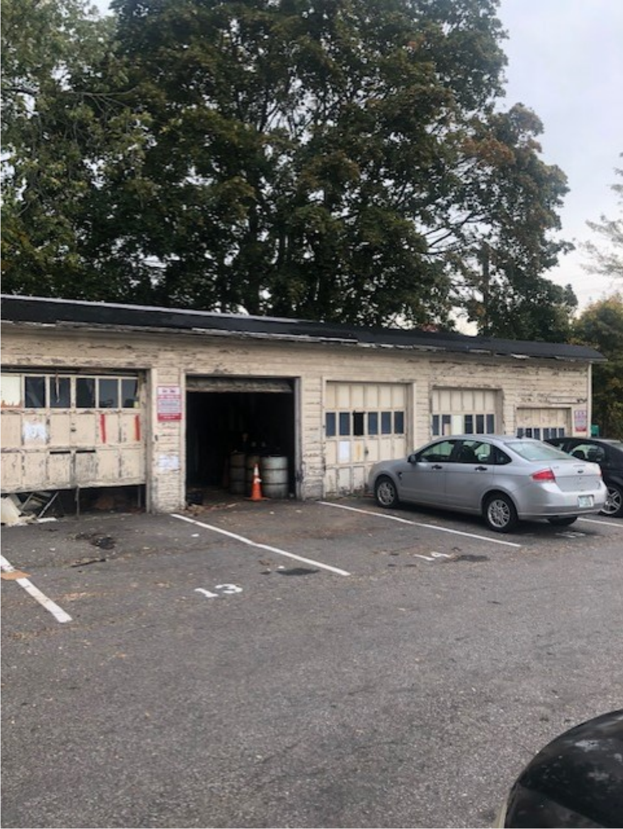
60-68 Wallingford Square Building – Existing Condition (Garage Portion #2)
