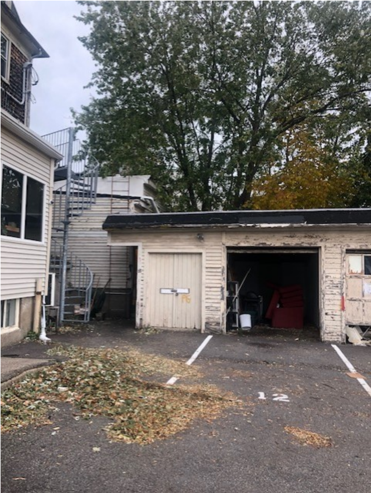
60-68 Wallingford Square Building – Existing Condition (Garage Portion #1)
