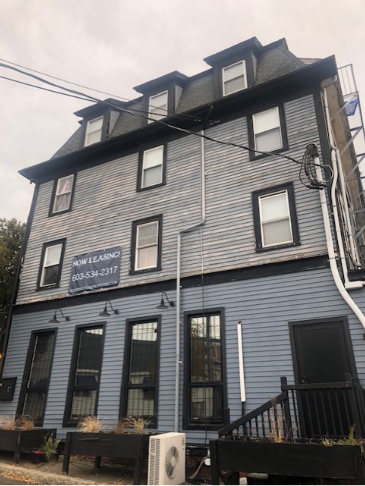
60-68 Wallingford Square Building – Existing Condition (Side Facade)
