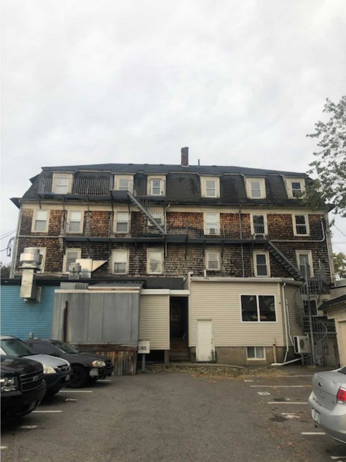
60-68 Wallingford Square Building – Existing Condition (Rear Façade)
