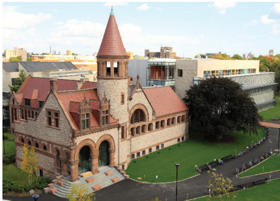
Honor Historically Significant Structures
