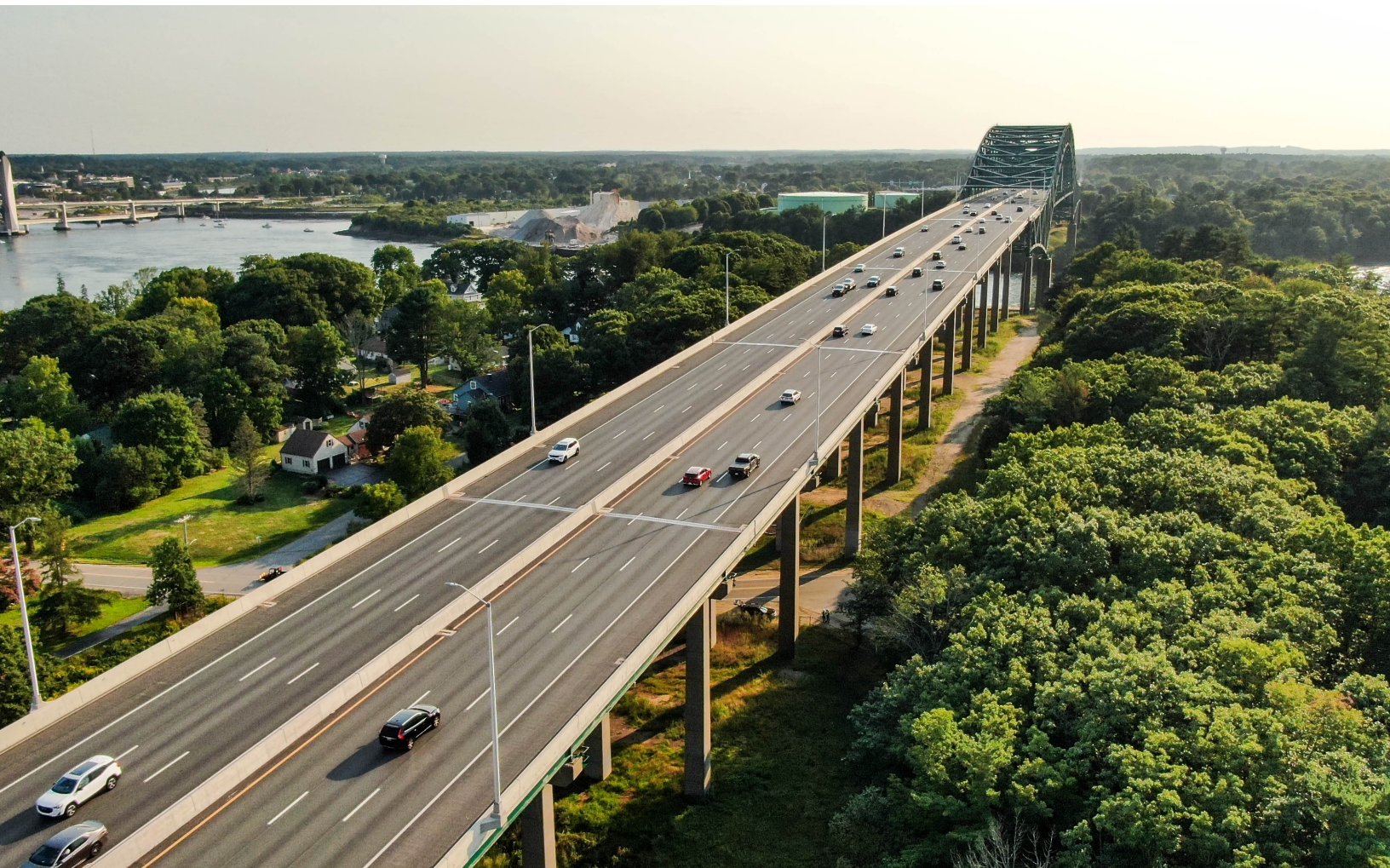
Piscataqua Bridge Rehabilitation
