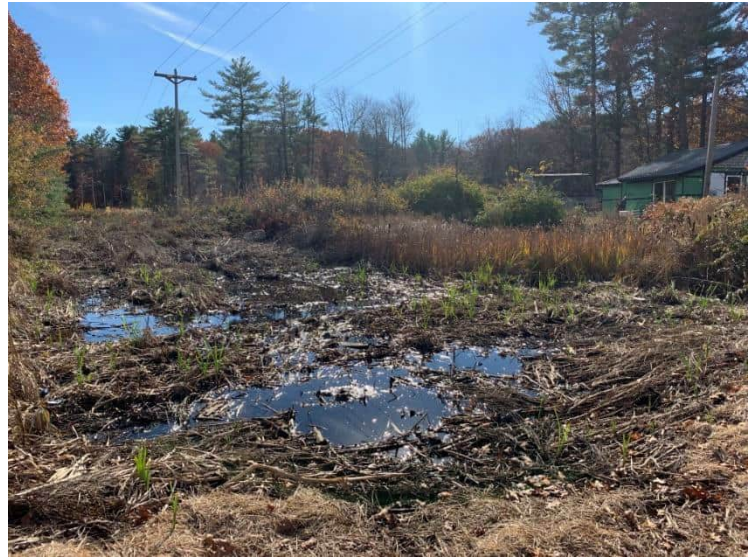
Photo 31. A view of the powerline right-of-way from Martin Road.
