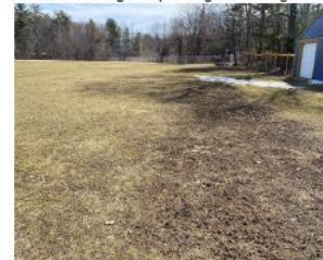
Photo 3: Large bare spots and evidence of significant ponding along the foul line of right field.
