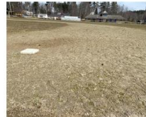
Photo 5: Poor condition infield that is saturated with evidence of ponding and moss growing.
