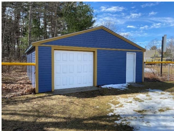
Photo 11: The existing storage building appears to be in good condition.
