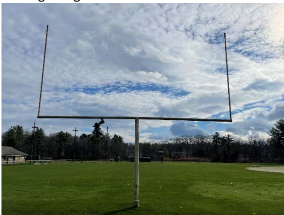
Photo 5: View of a rusty football goal post in poor condition.
