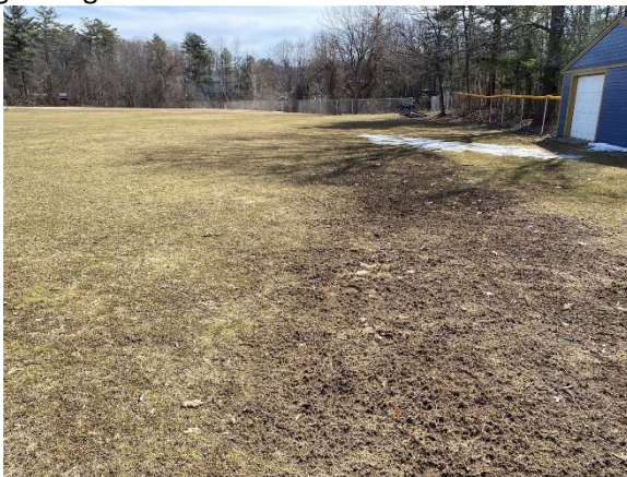
Photo 3: View of large bare spots and evidence of significant ponding along the foul line of right field.
