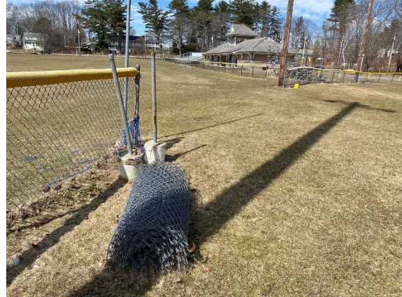
Photo 2: Centerfield fencing is partially temporary.
