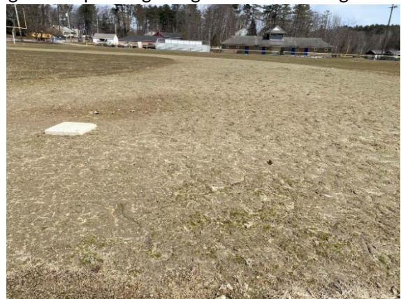
Photo 5: View of the poor condition of the infield, which is saturated and has evidence of ponding and moss growing.
