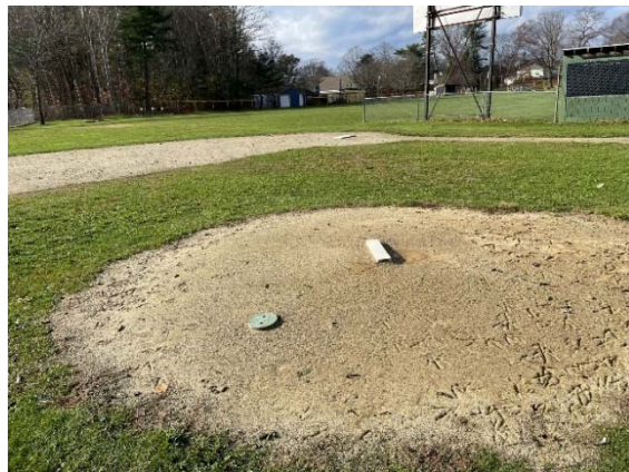
Photo 6: The pitcher's mound and infield are in fair condition. The irrigation valve is a tripping hazard.
