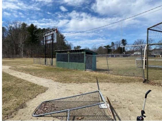
Photo 2: The dugout, fencing, equipment, and home plate all in fair condition; a hole was observed in home plate.
