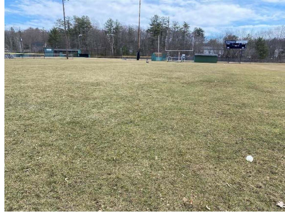
Photo 2: View of dips and heaves in the football field playing surface.
