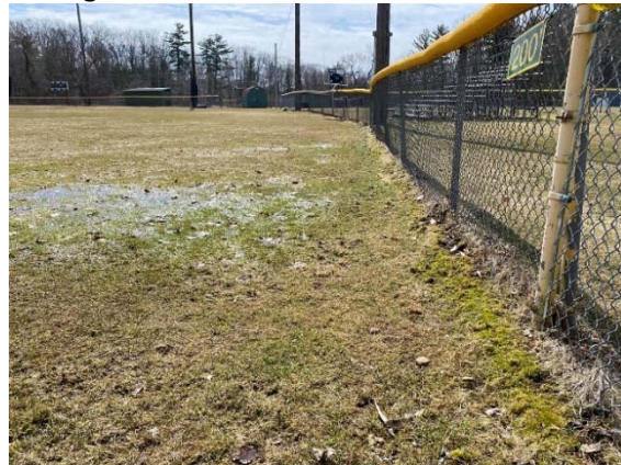
Photo 10: View of a depression in the corner of the outfield that results in significant ponding on the playing surface.
