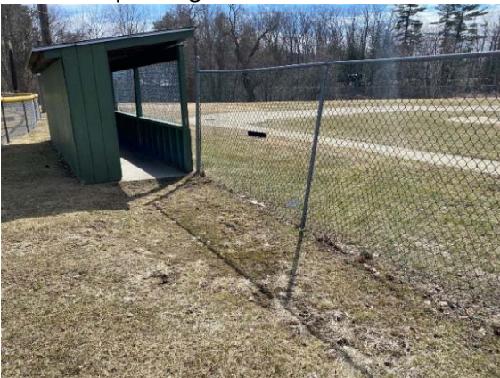
Photo 5: Fencing along the dugout is in fair condition, with bare spots/evidence of ponding.
