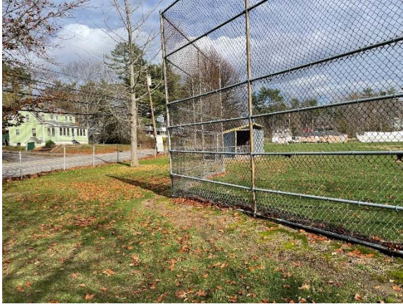
Photo 7: View of the old backstop, which is in fair condition with evidence of ponding.
