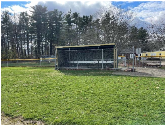
Photo 9: The right field dugout is in fair condition with bare spots and evidence of ponding.
