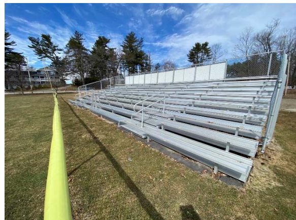
Photo 6: View of spectator seating with no accessible path or parking.
