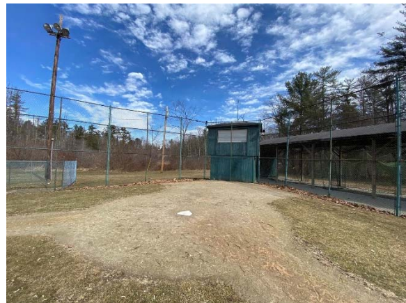
Photo 4: View of the backstop, press box, batter's circle, and athletic lighting.
