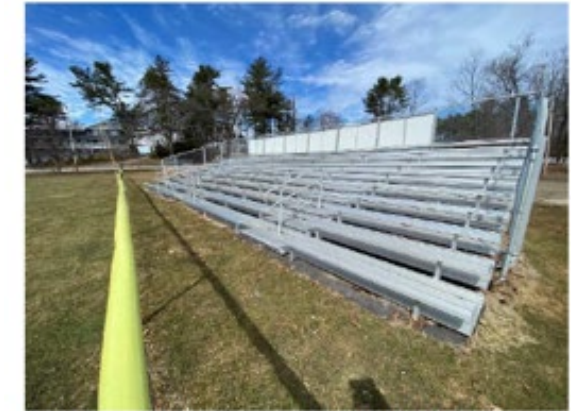
Photo 6: View of spectator seating with no accessible path or parking.
