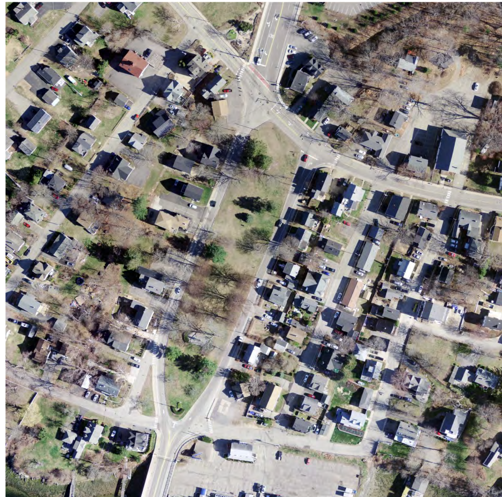
Figure 36: Existing Conditions – John Paul Jones Park
