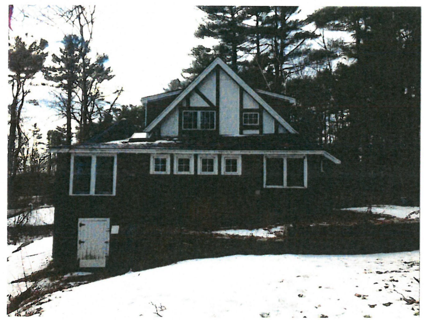
VIEW OF EAST SIDE ELEVATION
