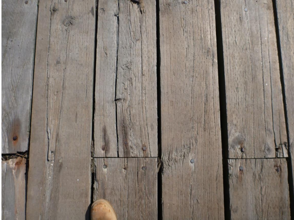
Figure 12 – Typical Condition of Decking
