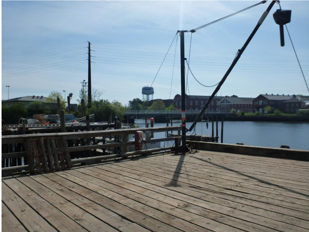
Figure 34 – Hoist located at southeast corner of pier
