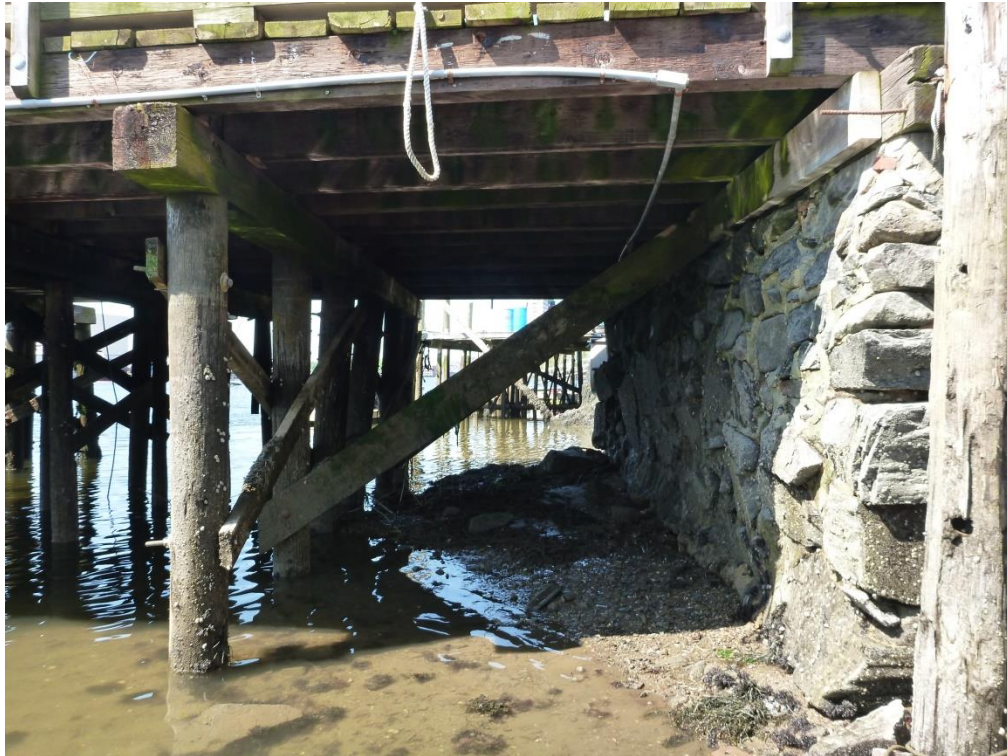
Figure 10 – View of bulkhead, pile supports, and bracing (Lines 4 & 5)
