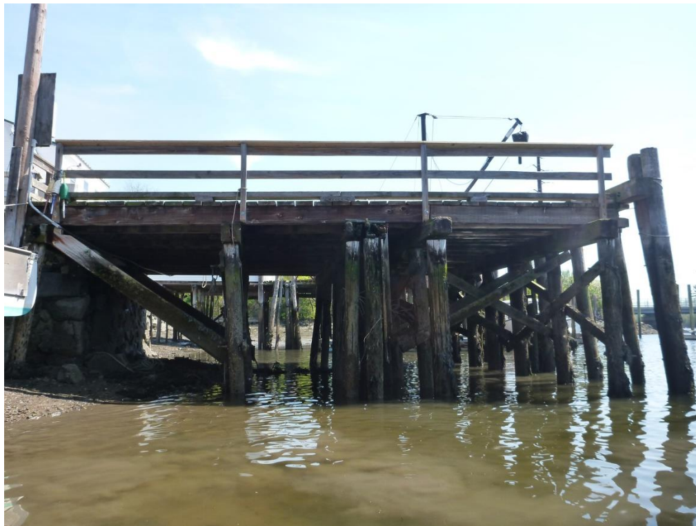
Figure 9 – West side of pier
