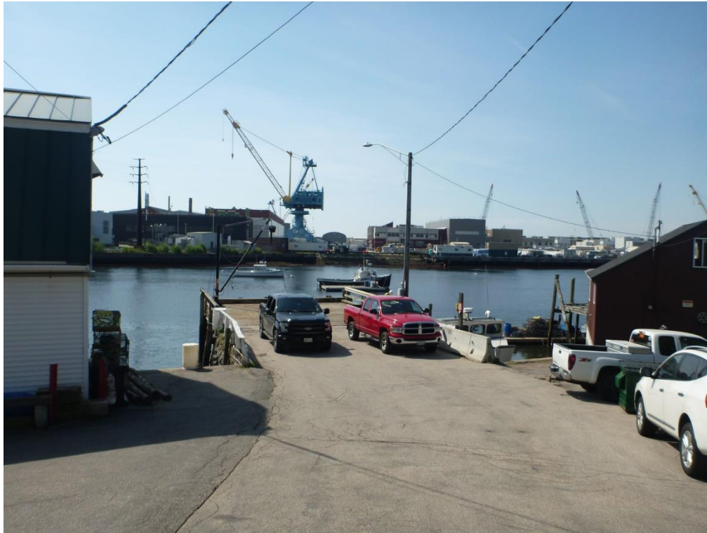
Figure 6 – View of Pier from Town Landing Road
