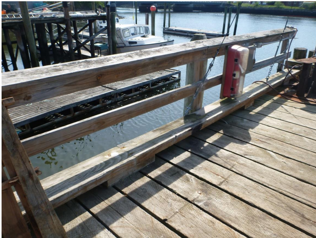
Figure 27 – Typical Railing and Curb on East side of pier
