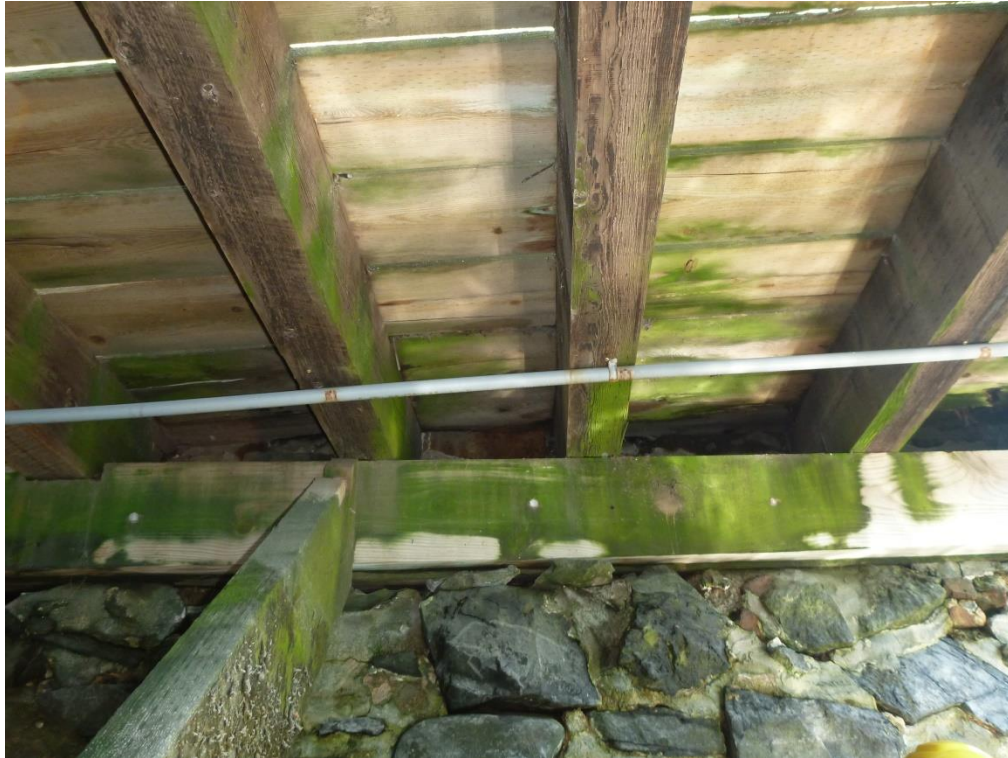
Figure 26 – Bent 5 pile cap supported on rock bulkhead
