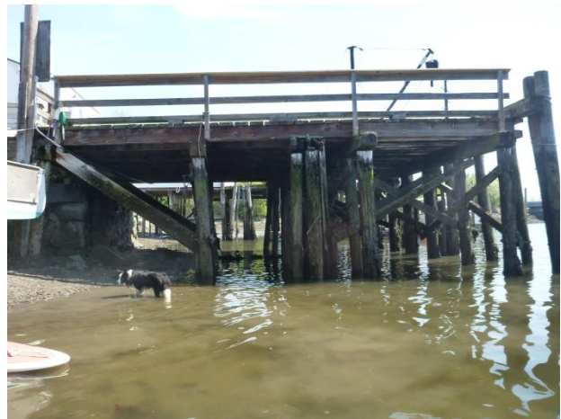
Figure 2 – View of East Side of Pier
