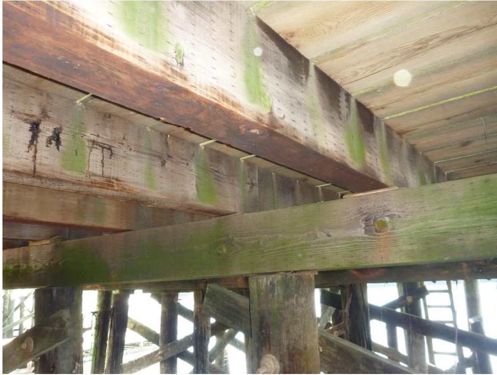
Figure 16 – Typical Condition of Stringers
