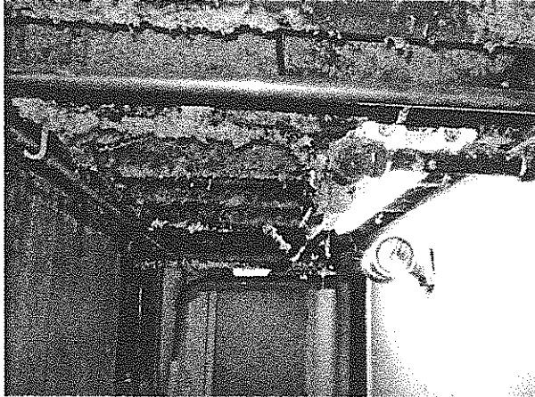
Blown-in insulation in Basement Hallway of 2 Walker Street Building.
