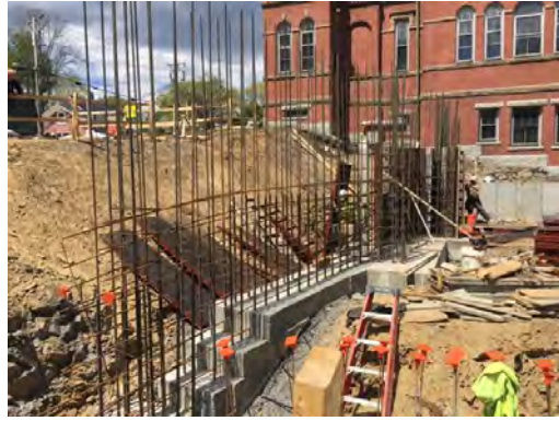
4. North side: footing below Community Rooms.
