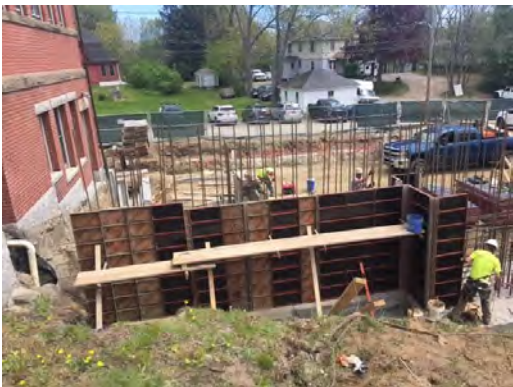
1. Northwest corner of addition: Forming foundation wall below new entrance.
