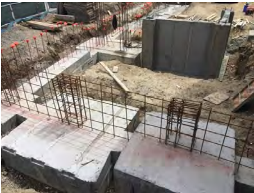
7. East side: footing below Maine Room and Collection.
