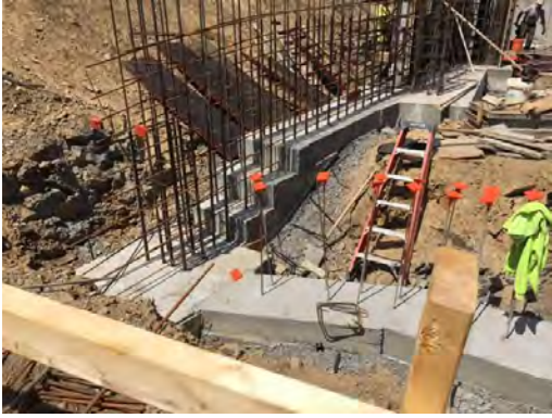
3. Northwest corner: footing below Community Room.
