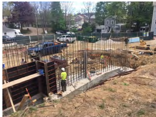
2. Northwest corner of addition: Footing below Community Rooms.
