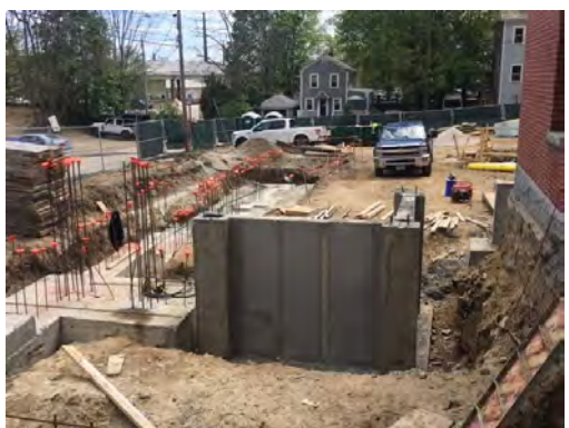
8. East side: Elevator shaft.
