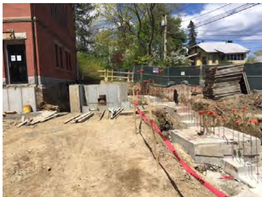
6. South side: Footing below toilets and stair.
