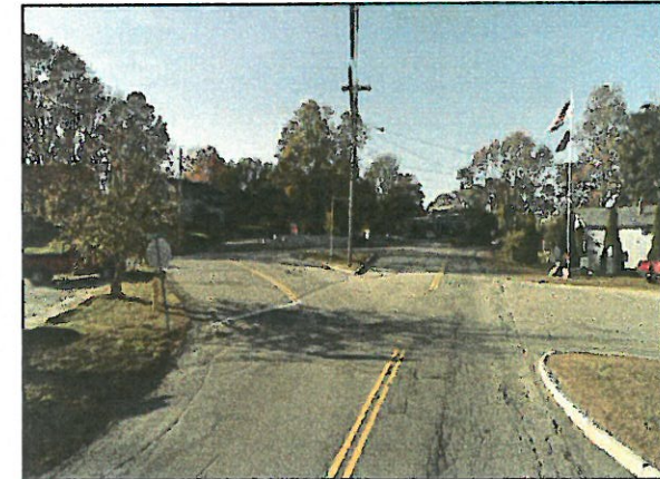
Intersection of State Road and Rogers Road, one of the high crash locations.
