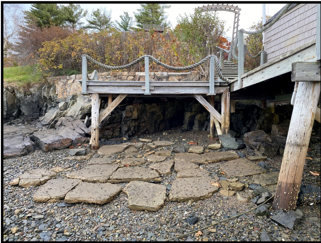
Photo 4. Existing Deck – Facing North from Intertidal Zone
