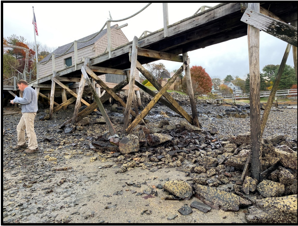
Photo 1. Existing Pier – Facing North from Intertidal Zone
