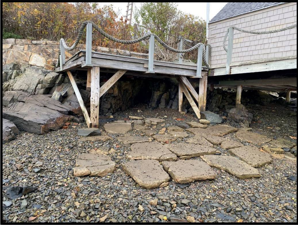
Photo 5. Existing Deck – Facing Northeast from Intertidal Zone
