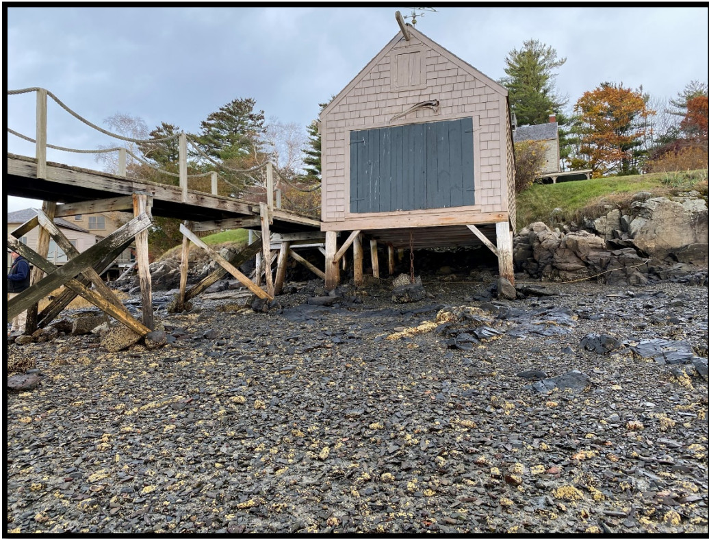
Photo 2. Existing Boat House – Facing North from Intertidal Zone
