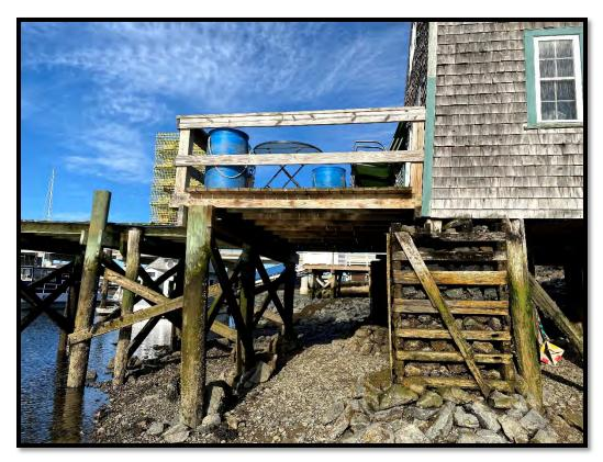
Photo 6. Seaward End of Boathouse to be replaced. Wharf to Remain.
