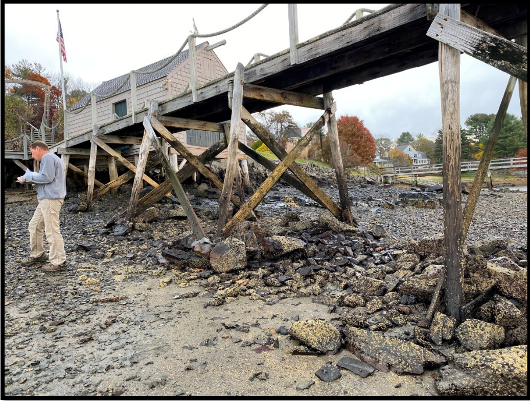
Photo 1. Existing Pier – Facing North from Intertidal Zone
