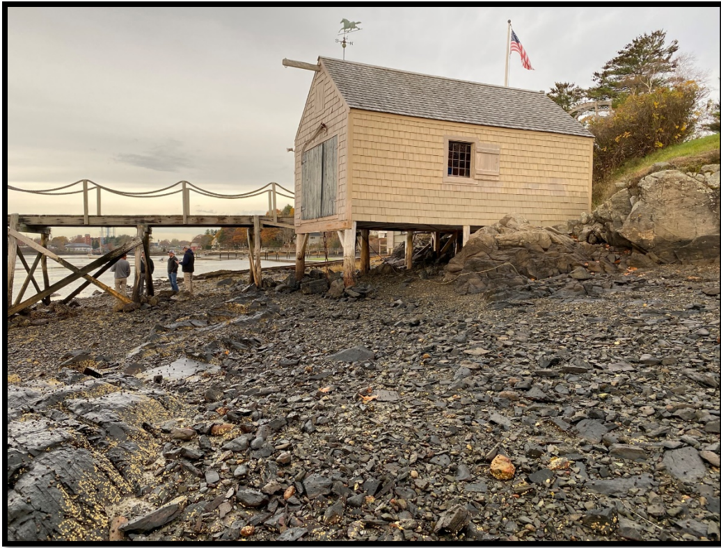
Photo 3. Existing Pier and Boat House – Facing West from Intertidal Zone
