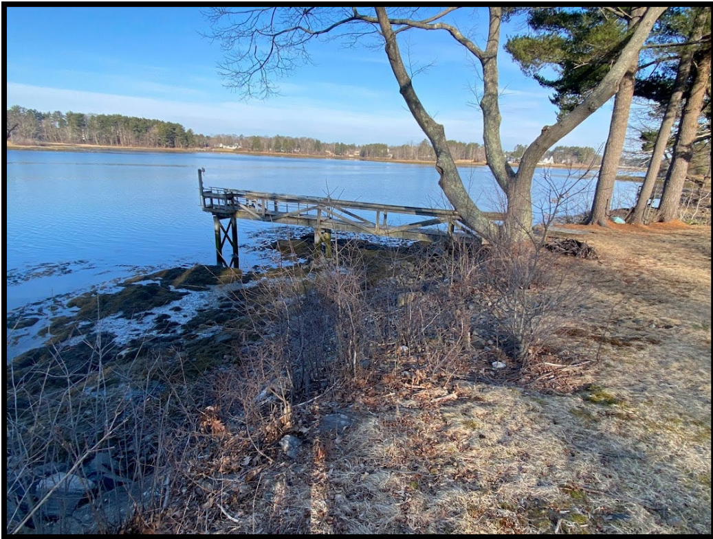
Photo 2: Existing Pier Structure Facing Northwest
