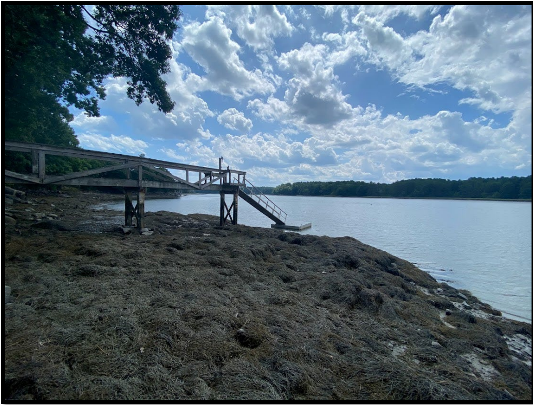
Photo 3: Existing Pier Structure Facing Southwest
