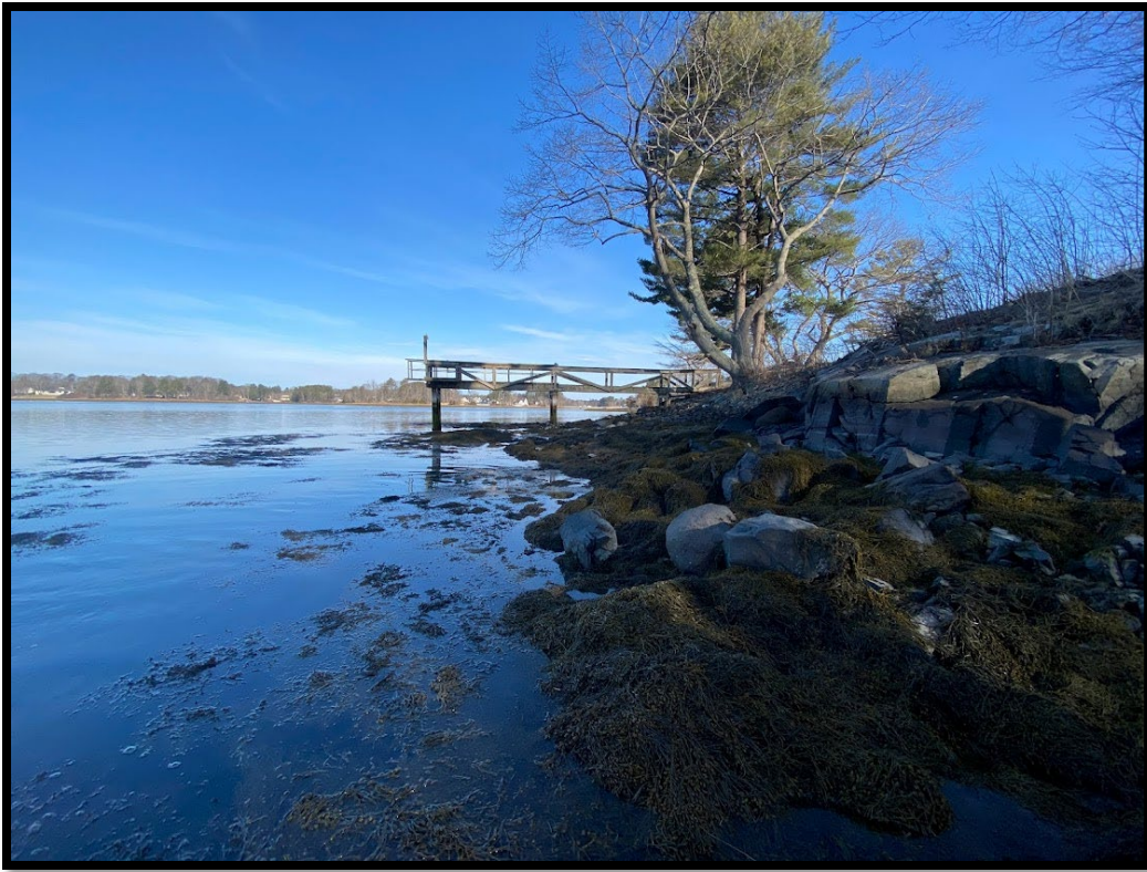
Photo 1: Existing Pier Structure Facing North
