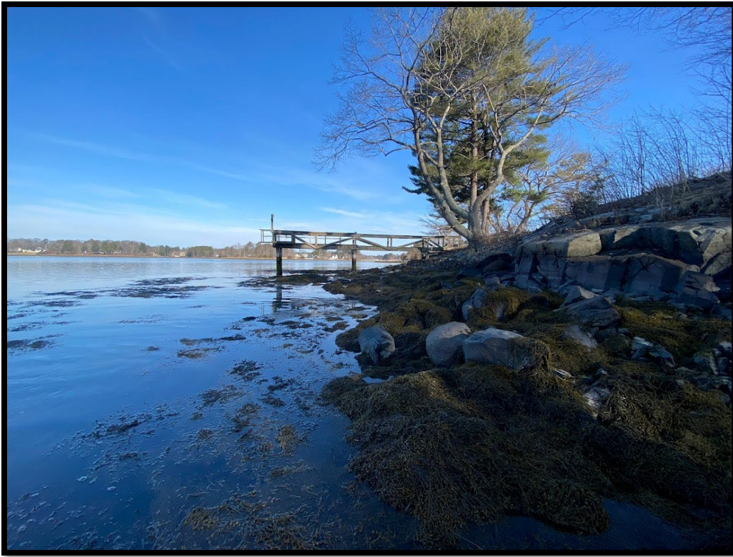
Photo 1: Existing Pier Structure Facing North
