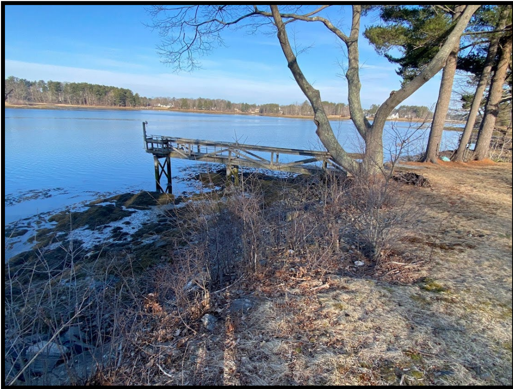
Photo 2: Existing Pier Structure Facing Northwest
