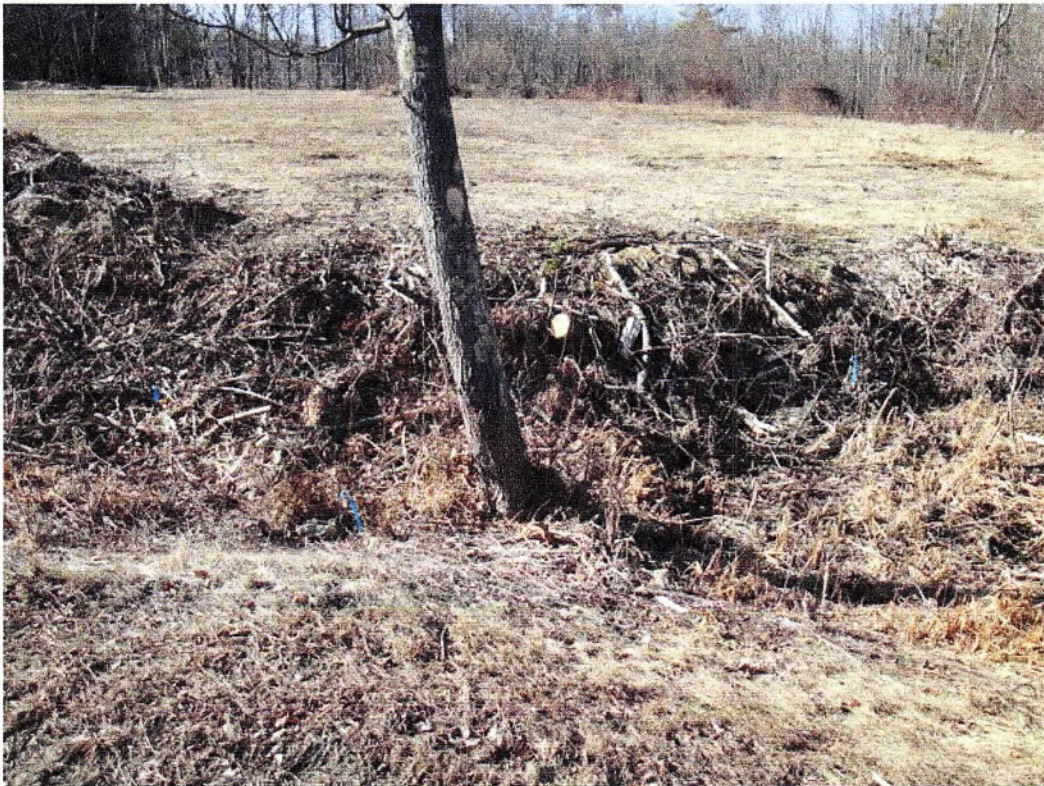
Another View Of The Wetland Area That Meets The Local Definition Of A Drainage Ditch
