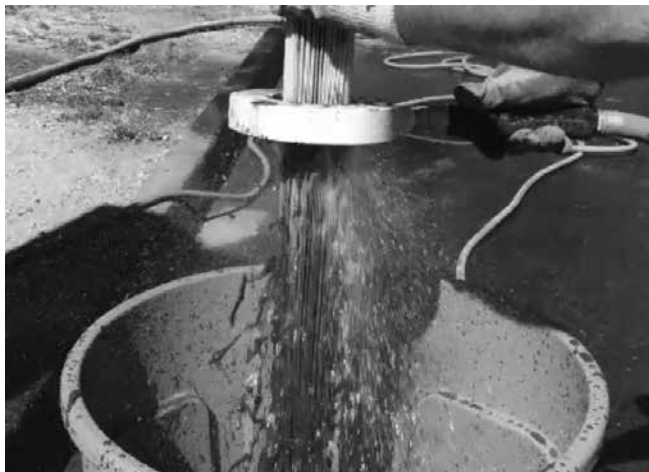
Vacuuming Sump Through MAW
