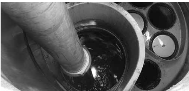
Vacuuming Sump Through MAW
