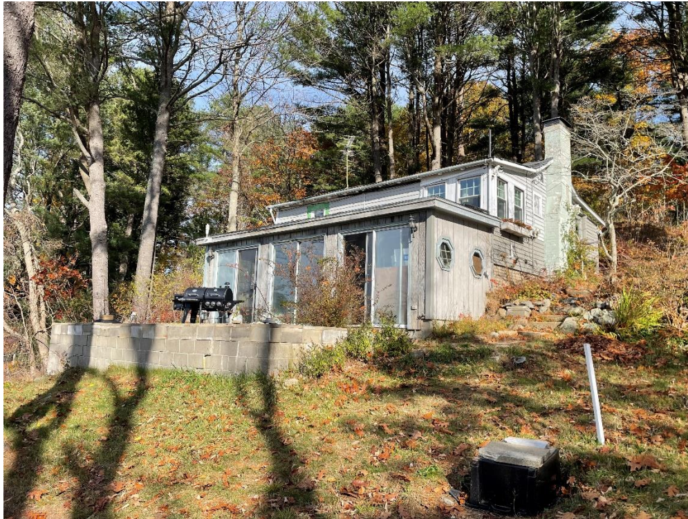
South Side of Main House
