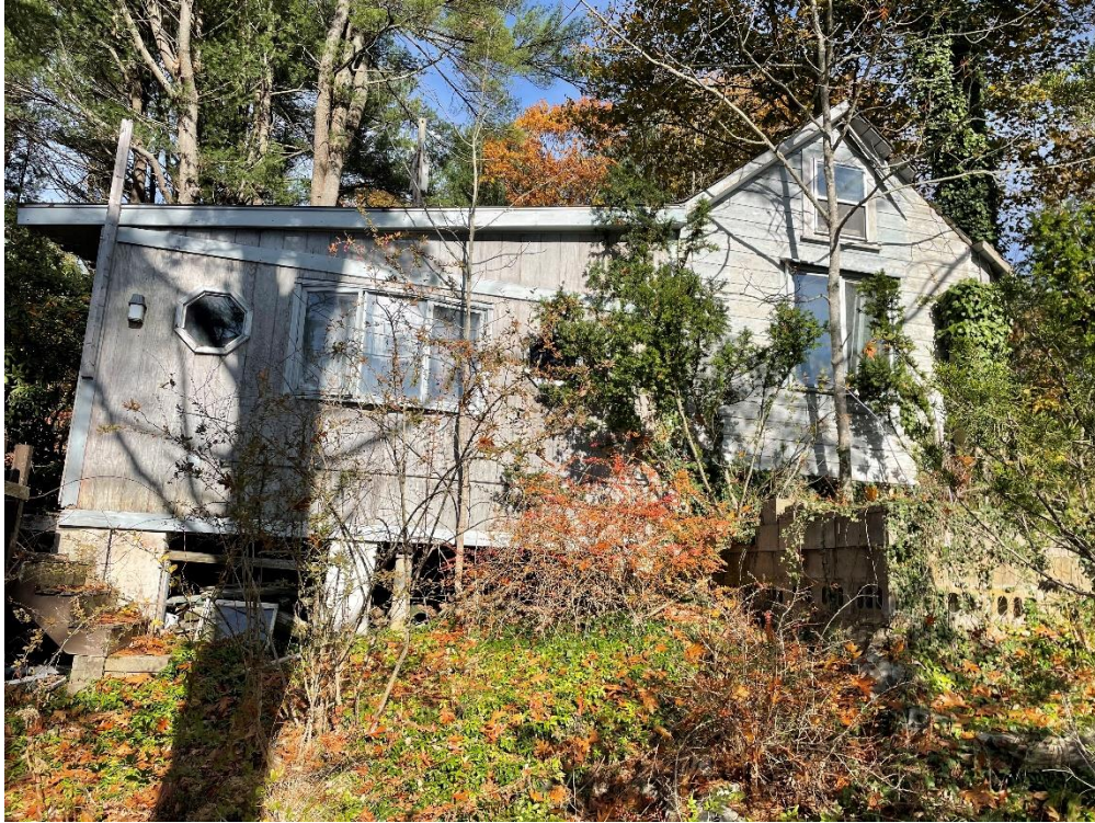
Southeast Side of Garage/Guest House
