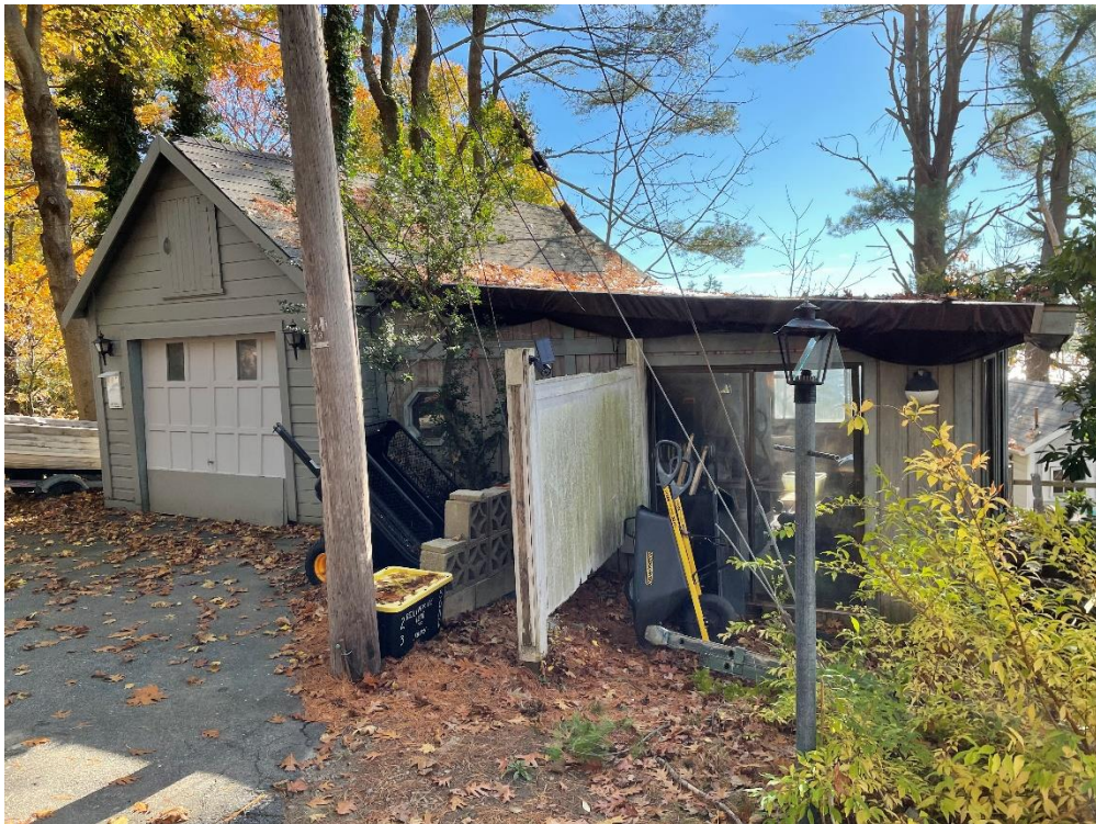
Northeast Side of Garage/Guest House
