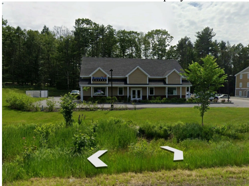
Photo #2: Front of Property
