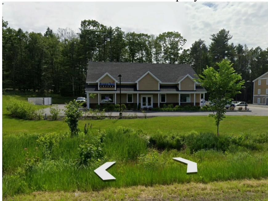
Photo #2: Front of Property
