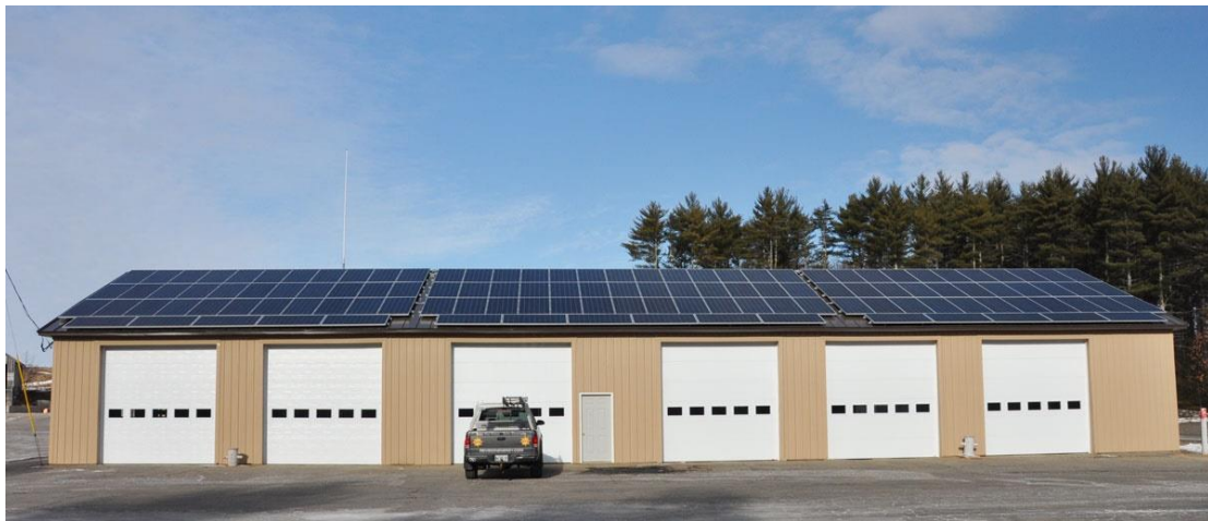
Solar panels on the roof of the Wells Town Garage reduce municipal electricity emissions and produce utility cost savings.
