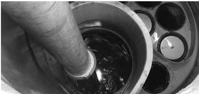
Vacuuming Sump Through MAW
