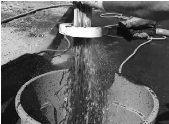
Vacuuming Sump Through MAW
