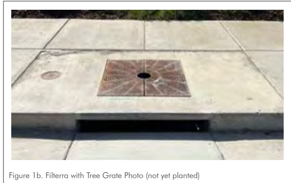
Figure 1b. Filterra with Tree Grate Photo (not yet planted)
