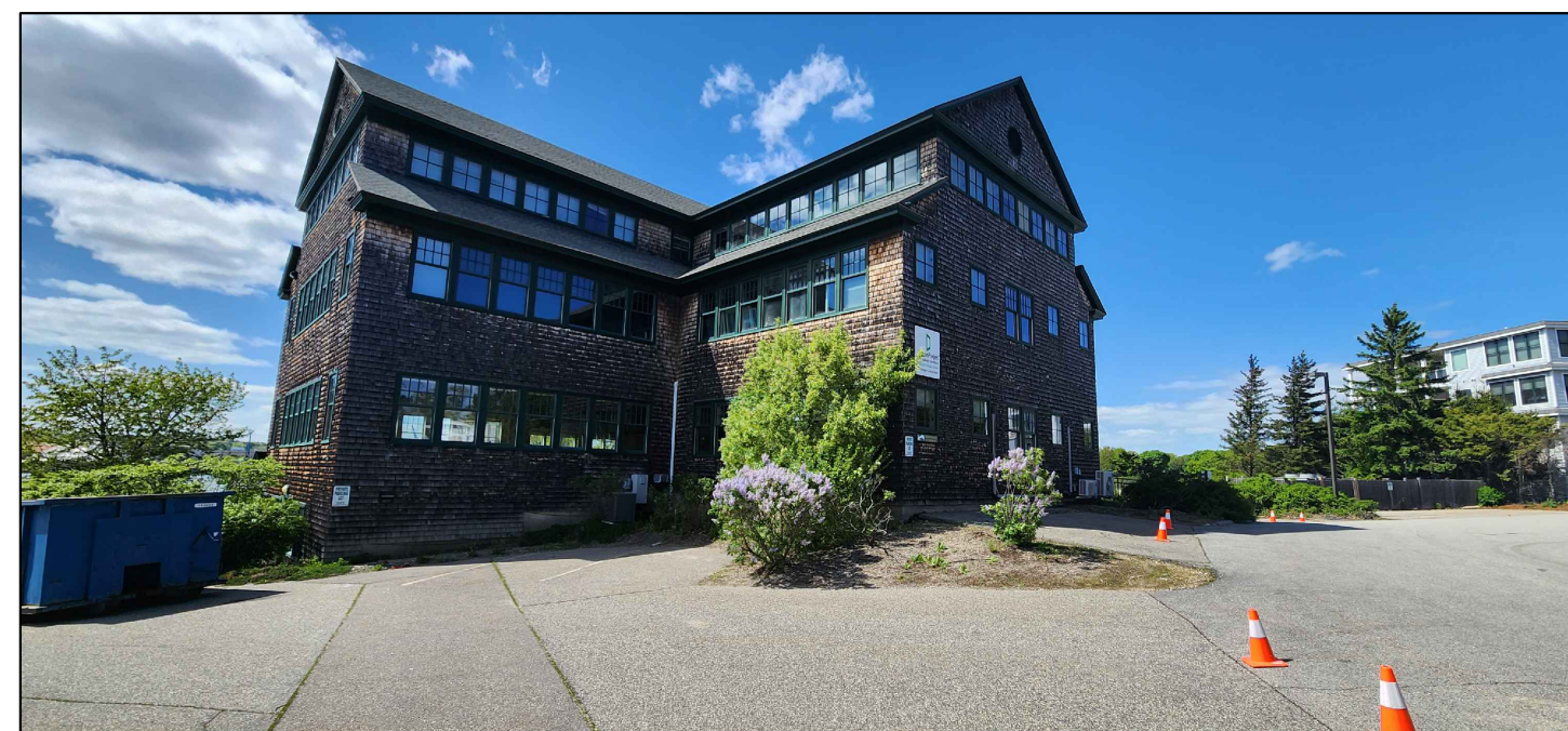
35 BADGERS ISLAND WEST - PROJECT SITE
