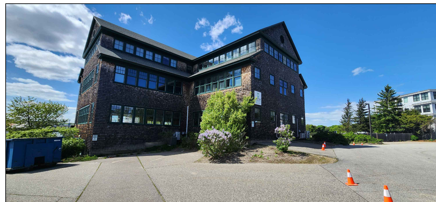
35 BADGERS ISLAND WEST - PROJECT SITE
