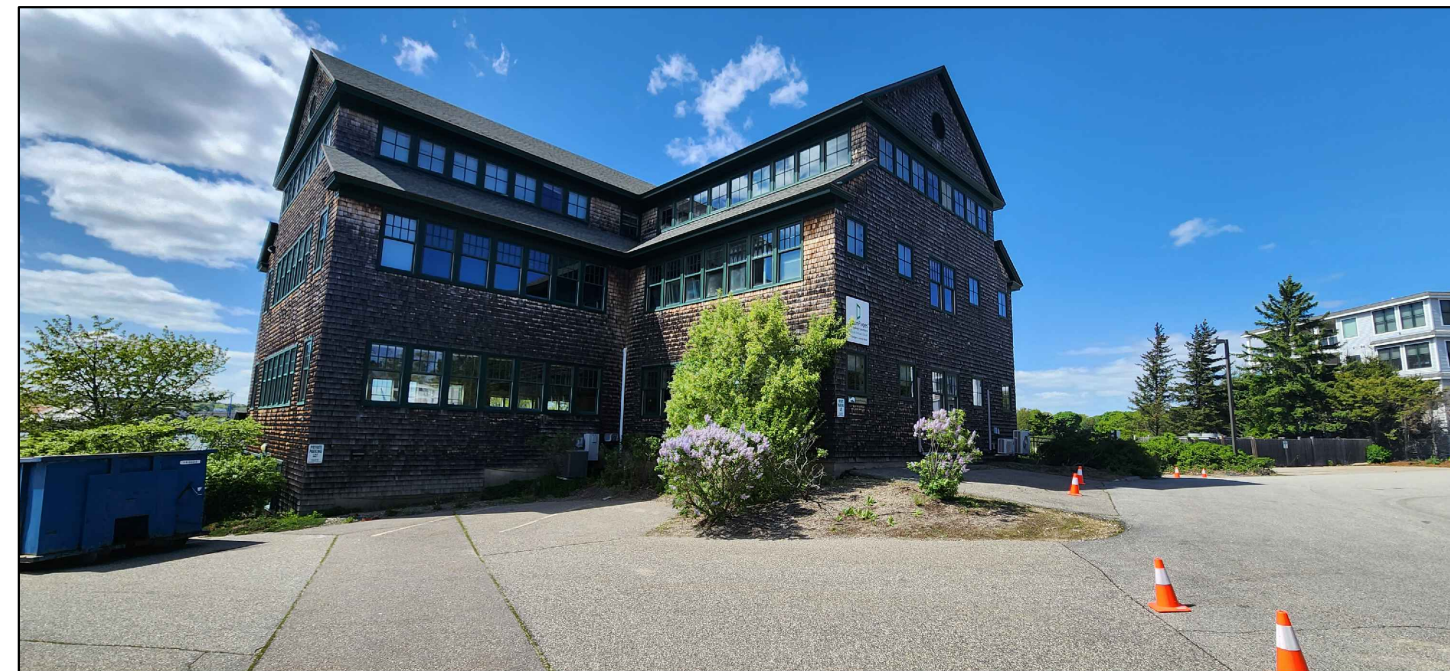
35 BADGERS ISLAND WEST - PROJECT SITE
