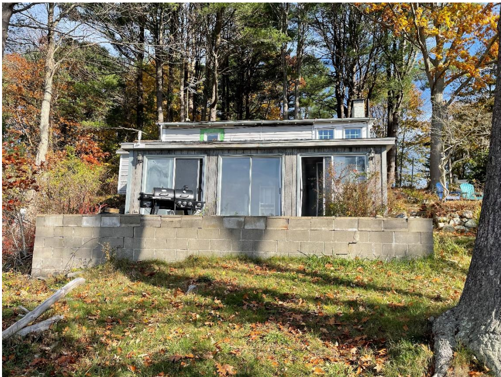
View of Main House from Spruce Creek
