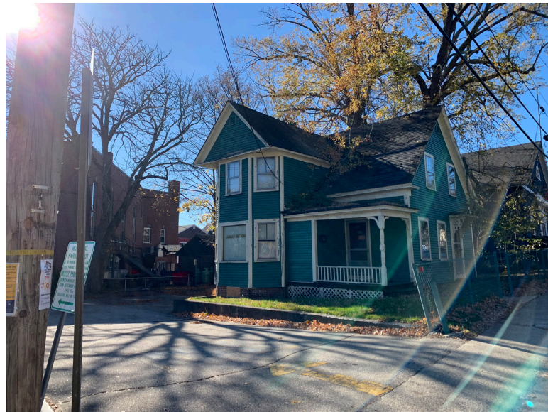
IMAGE 1: SITE - LOOKING SOUTHWEST
