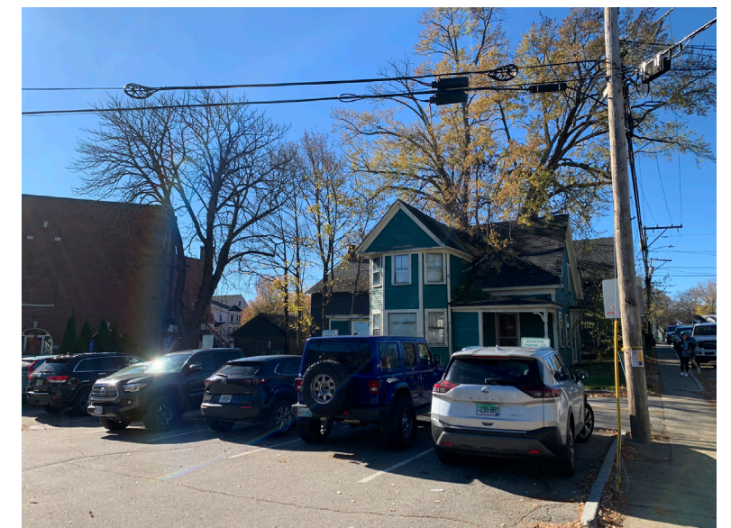
IMAGE 6: SITE - LOOKING SOUTHWEST
