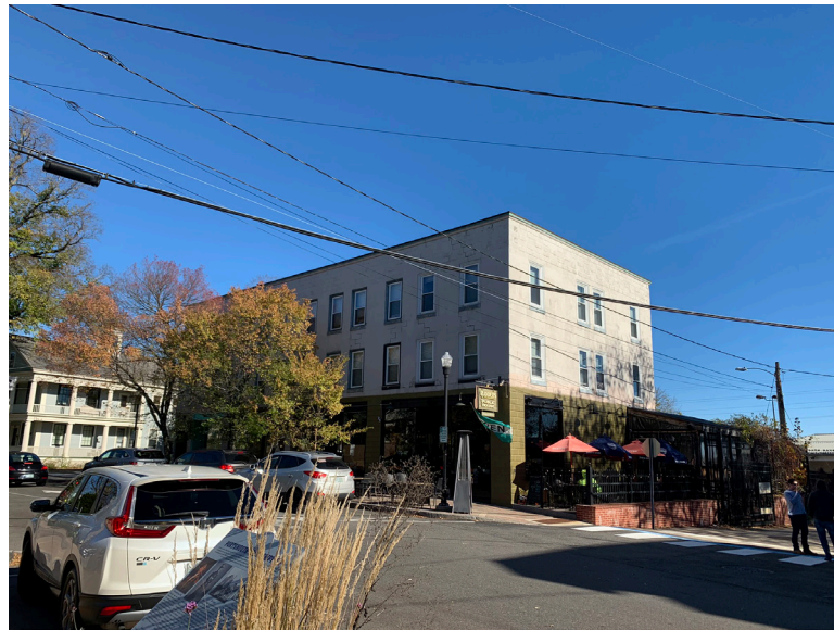
IMAGE 4: 70-78 WALLINGFORD SQUARE BUILDING
