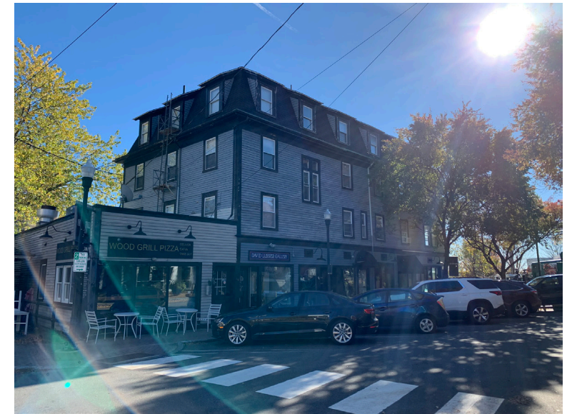
IMAGE 5: 60-68 WALLINGFORD SQUARE BUILDING
