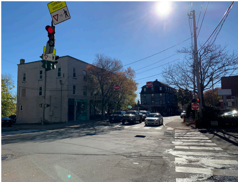
IMAGE 3: 70-78 WALLINGFORD SQUARE BUILDING
