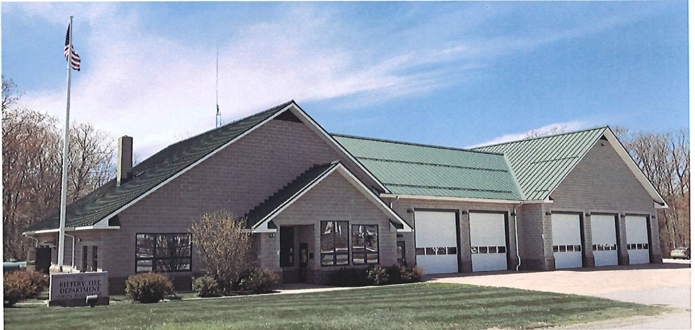
Existing Northeast View
