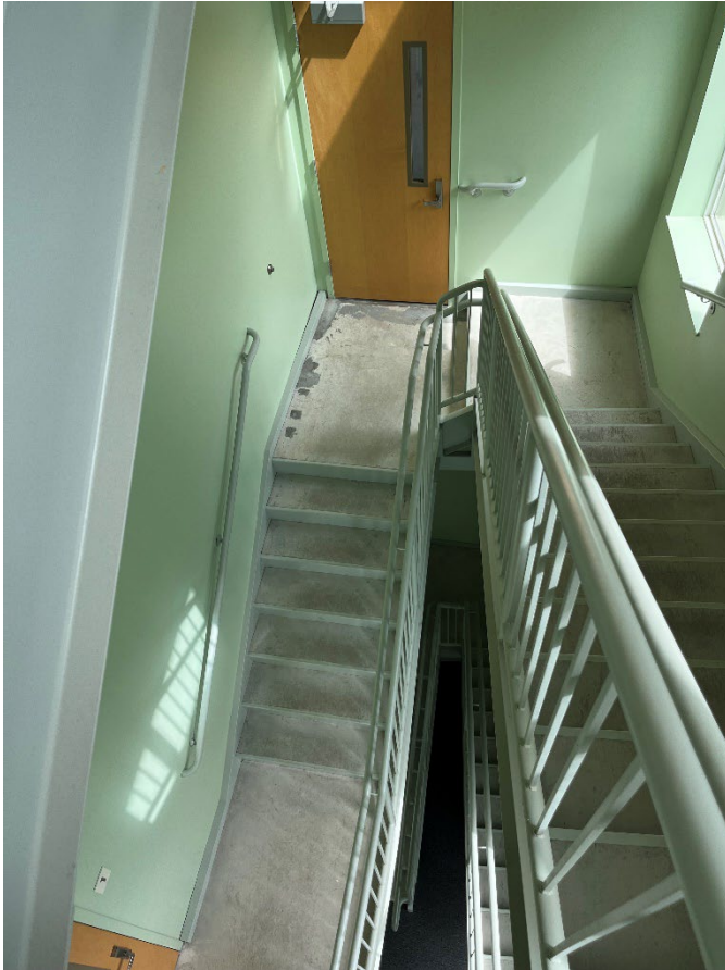
c. Sealed concrete floor in the stairwell A is spotty and cracking
