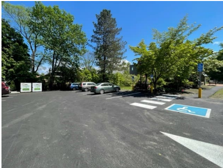
1. Upper parking lot with topcoat and painted.
