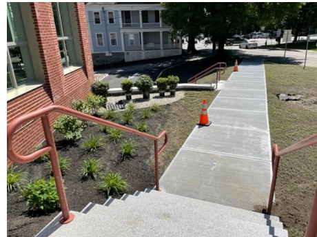
2. Sidewalk completed to Wentworth and landscaping along front of building.
