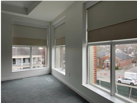
5. Window shades have been installed.
