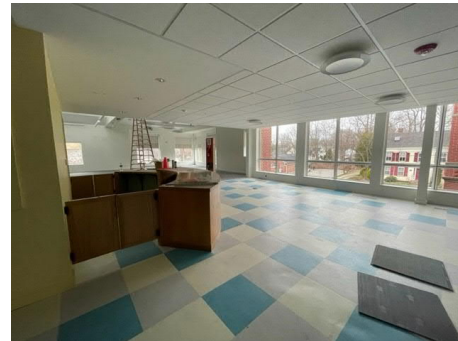
6. Flooring is completed with the exception of the lower level.
