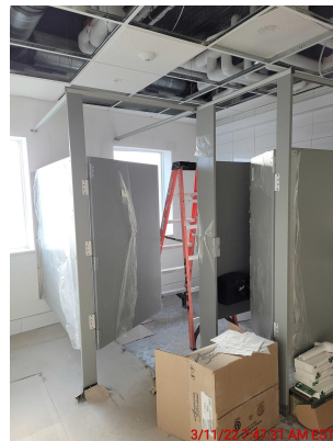
4. Ceiling tile and toilet partitions in progress.
