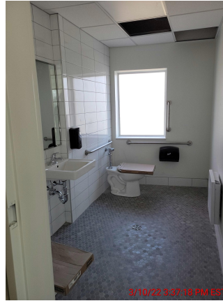
2. Restroom fixtures being installed.
