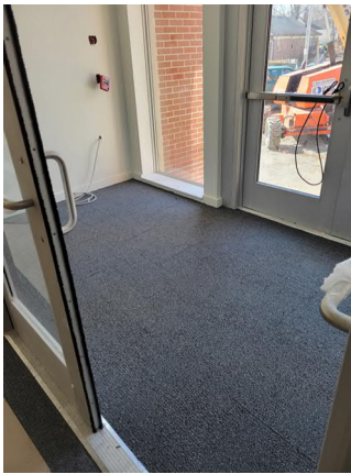
1. Front Entrance finishes In progress.
