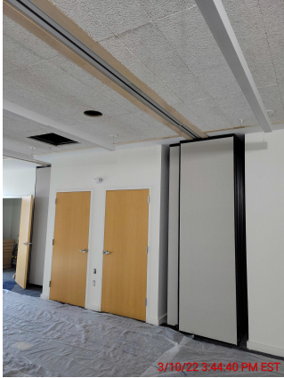
5. Folding Partitions in progress
