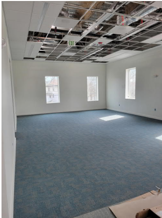
7. Ceiling tile and carpet in progress.
