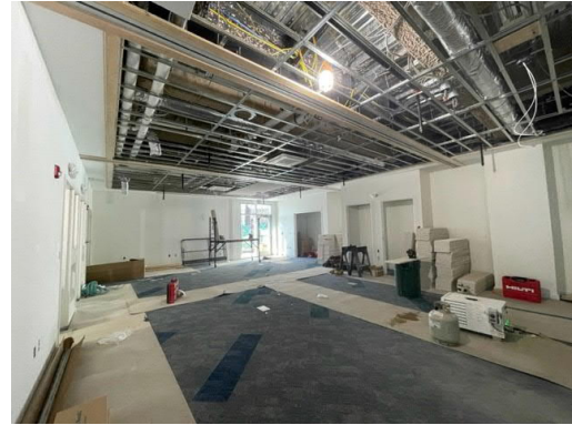
6. Carpet in progress in Lower Level.
