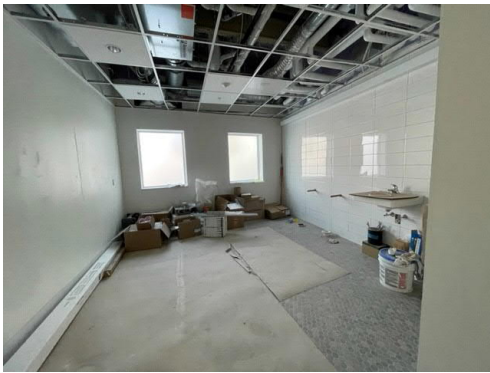
7. View of Restroom tiling.
