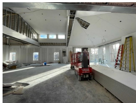
4. Drywall work in progress on 2 nd floor.
