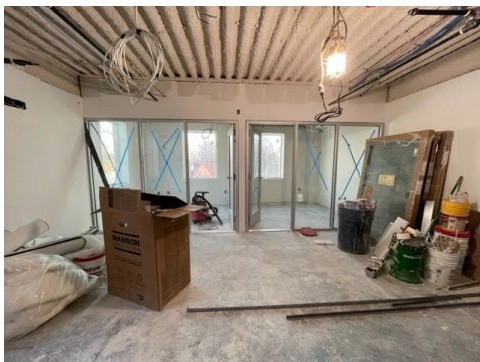
3. Doors and frames being installed.
