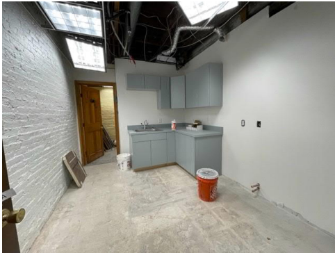
5. Staff Room Millwork and priming in Progress.
