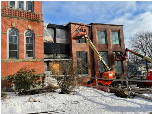
1. Windows at front façade being installed.
