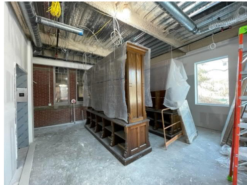
2. Existing bookcases relocated to the new Building.
