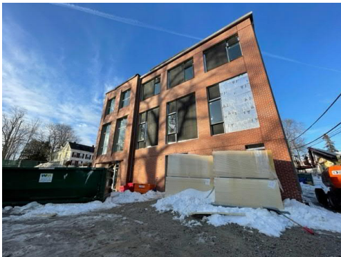
9. View of Traip Ave façade awaiting panels.
