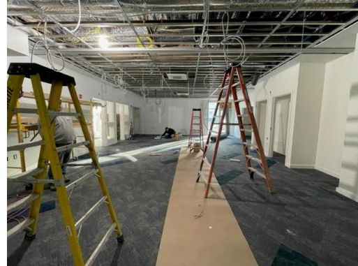
6. Carpet in progress in Lower Level.
