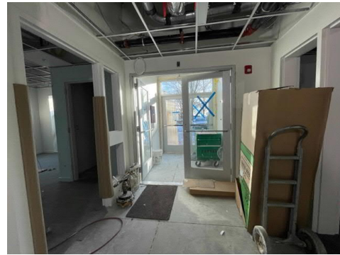
8. Exterior doors in progress.
