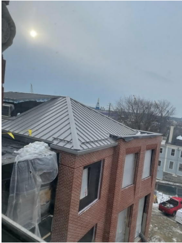
3. View of standing seam metal roof over the Children's Collection.
