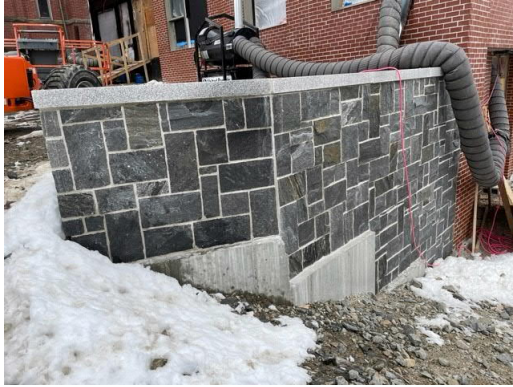
9. View of new retaining wall with granite veneer.
