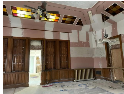
2. Patching in Existing Building, Reading Room.
