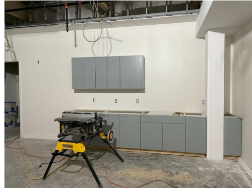
10. View of Lower Level Maker Space Millwork in progress.
