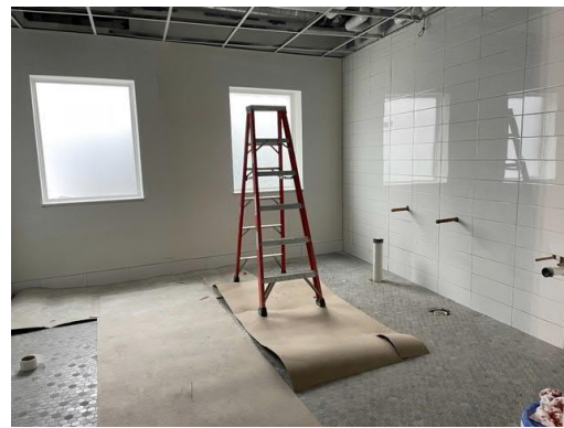
6. Lower Level restroom tiling in progress.
