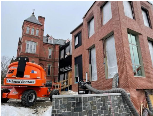
1. View of library from south showing new retaining wall.
