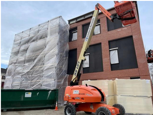
1. Brick work in progress on north façade.
