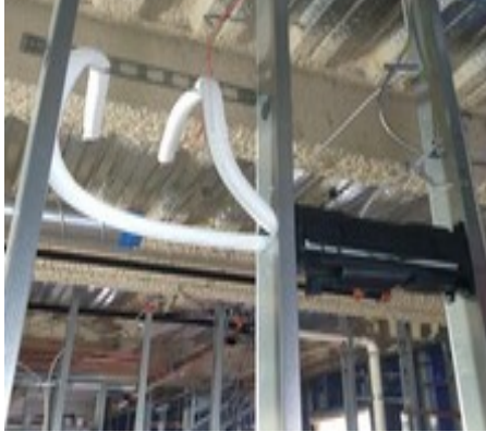
Figure 1: Fan Coil Unit Piping
