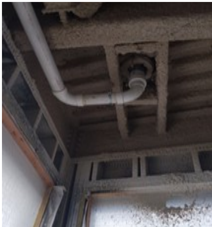
Figure 3: Corner Roof Drain
