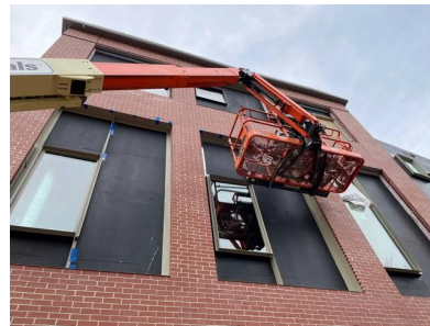
2. Brick work in progress on south façade And windows being installed.
