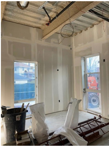
5. View of the Lower Level Meeting Room with drywall complete.
