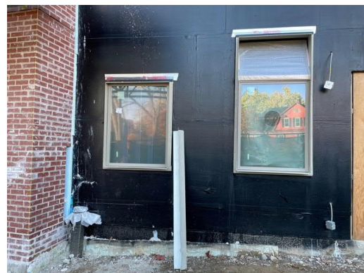
8. View of window installation in progress.
