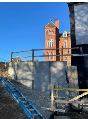
7. View of retaining wall concrete.
