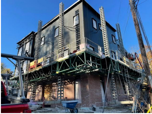
9. View of brick work in progress facing Traip Ave.
