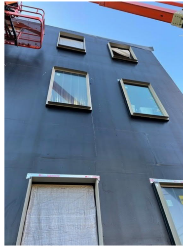
10. Another view of window install in progress.
