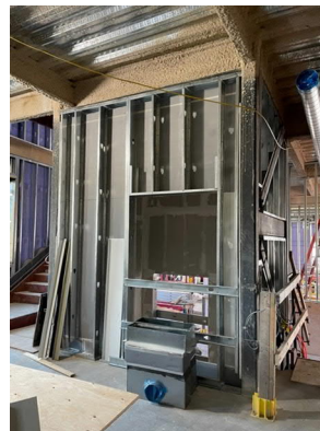
2. Framing of elevator shaft.
