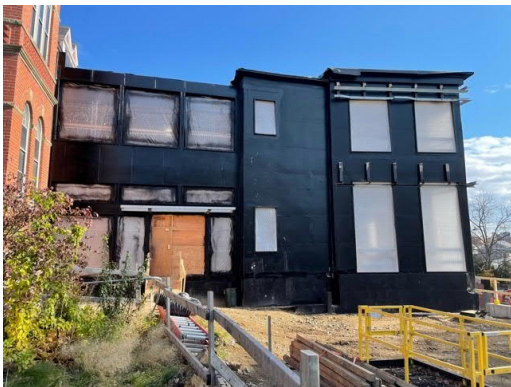
1. Vapor barrier done and windows with poly Installed over window openings.
