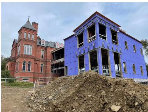
1. Overall Structure, view of sheathing in progress.
