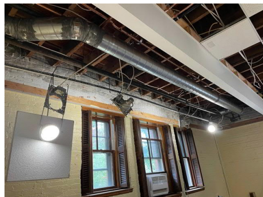
2. View of the existing building, lower level rough mechanical in progress.
