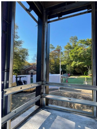
5. View from the first floor looking out towards the Taylor Building.
